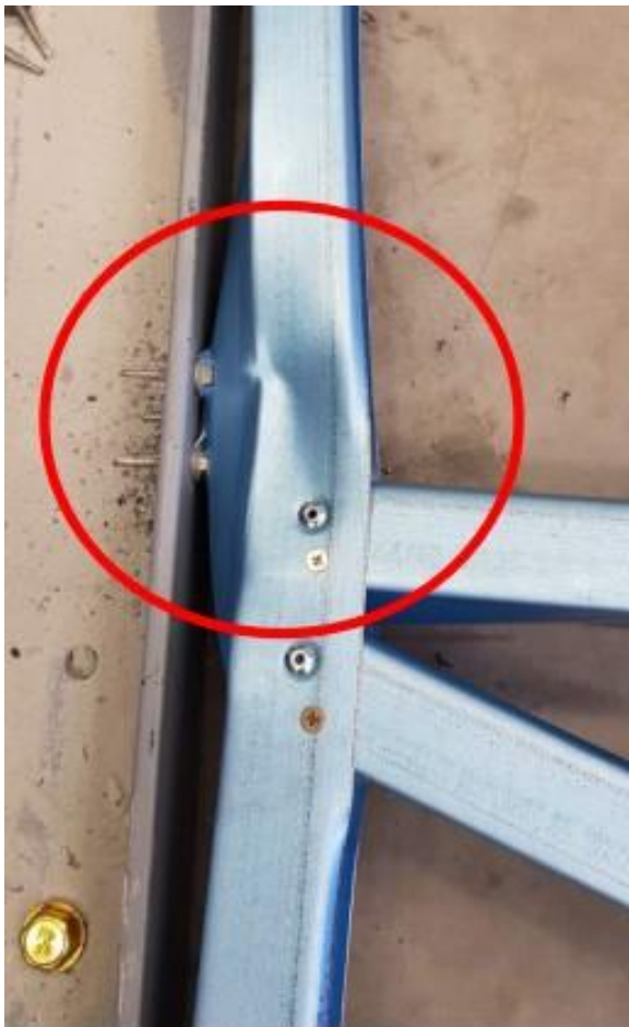
450mm K-BRACING CONNECTION
